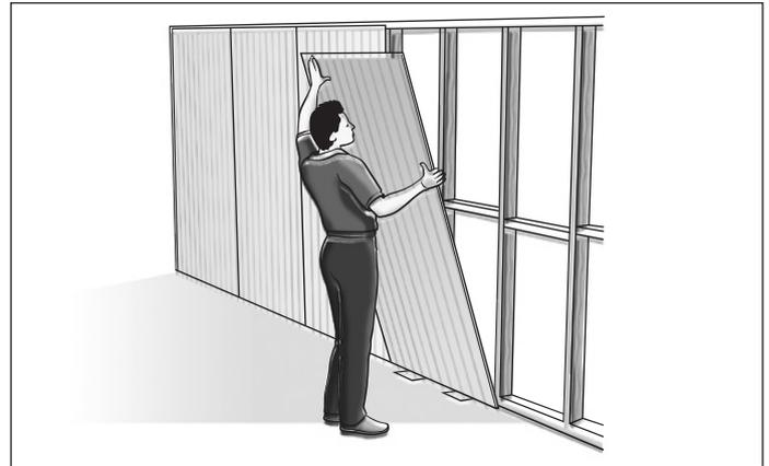
FIGURE 4 SHEET INSTALLATION
