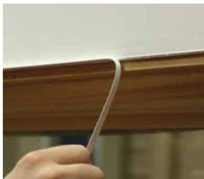
“ Protect adjoining surfaces while leaving a clean, finished edge with Trim-Tex Tear Away™ beads ”
