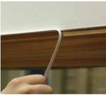
Protect adjoining surfaces while leaving a clean, finished edge with Trim-Tex Tear Away™ beads
