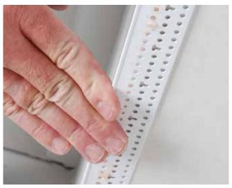
**3.** Apply firm, even pressure to the mud legs of the trim to ensure a solid bond
