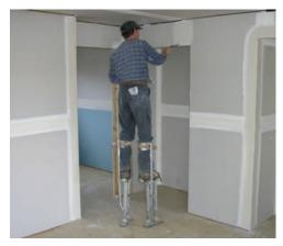
Correct use of stilts: A light duty task being conducted on a clean floor.
