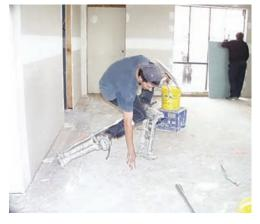
Inappropriate activity whilst on stilts: Reaching below foot level stresses the knee, ankle, back and stilts.
