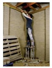
Inappropriate environment for working on stilts: Working in garage with earth floor and poor housekeeping.
